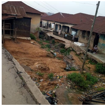
Plate D: Gully erosion aided by the geologic setting (Steepy terrain)
