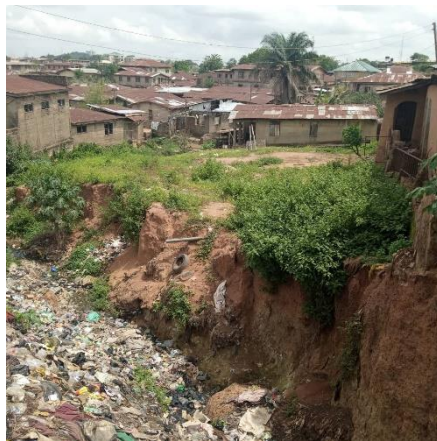
Plate C: A landscape chopped by gully erosion
