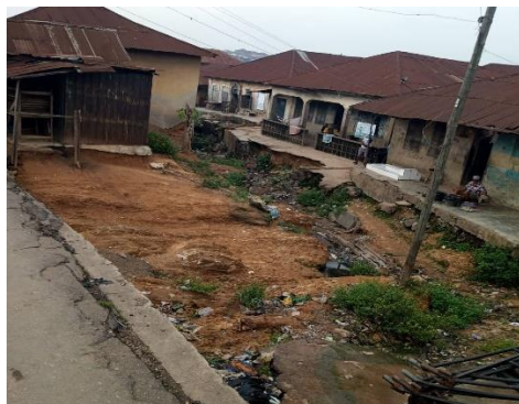
Plate A: Open space opposite residential homes gradually becoming gully due to surface runoff at Idi-Arere
