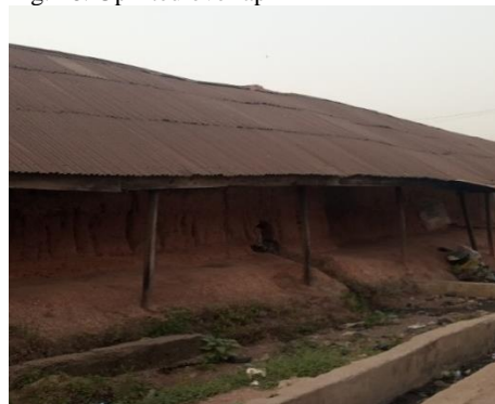
Fig. 19. Exposed Wall and Rustic Roof
