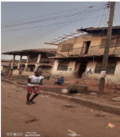
Fig. 15. Peeled Paint, Falling Roofing & Hanging Facial
