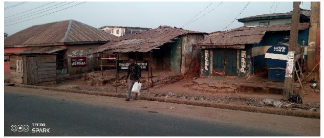
Fig 7. Up Lifted Overlaps
