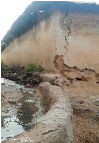
Fig 5: Wall Cracks
