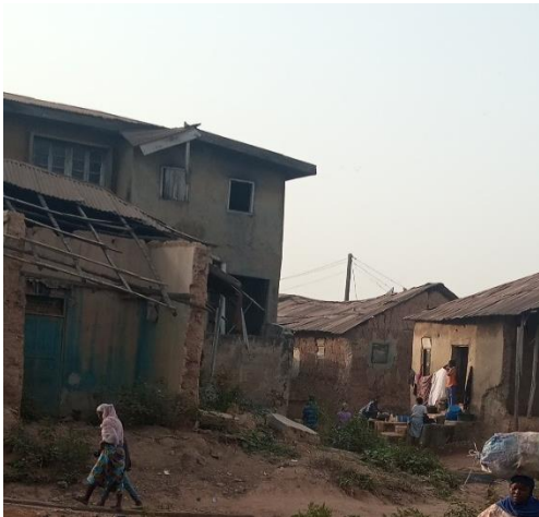
Fig 20. Hanging walls, loose door and window
