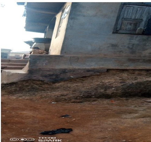
Fig. 22. Exposed foundation
